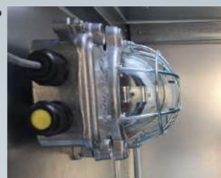
Explosion proof lamp For eliminate risk of explosion, all possible spark equipment shall be minimize risk of explosive.
